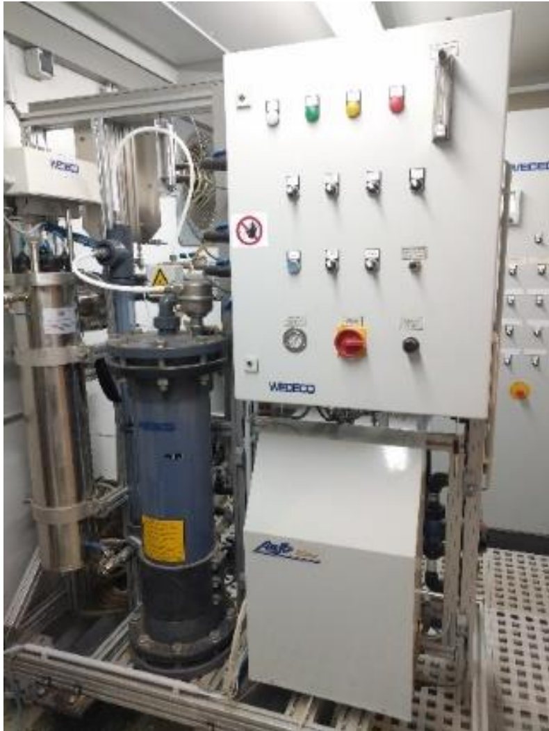
< Xylem WEDECO 8HC Ozone generator and UV reactor >
